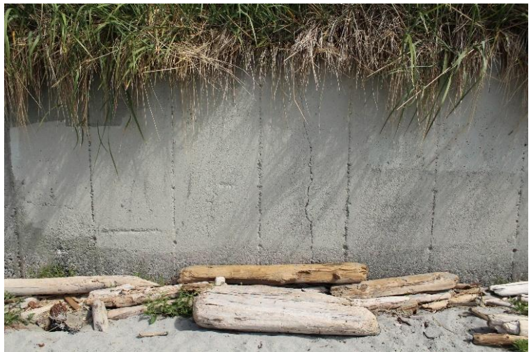
Figure 5 - An example of a seawall (one type of shoreline modification). Photo by Maria Catanzaro.
